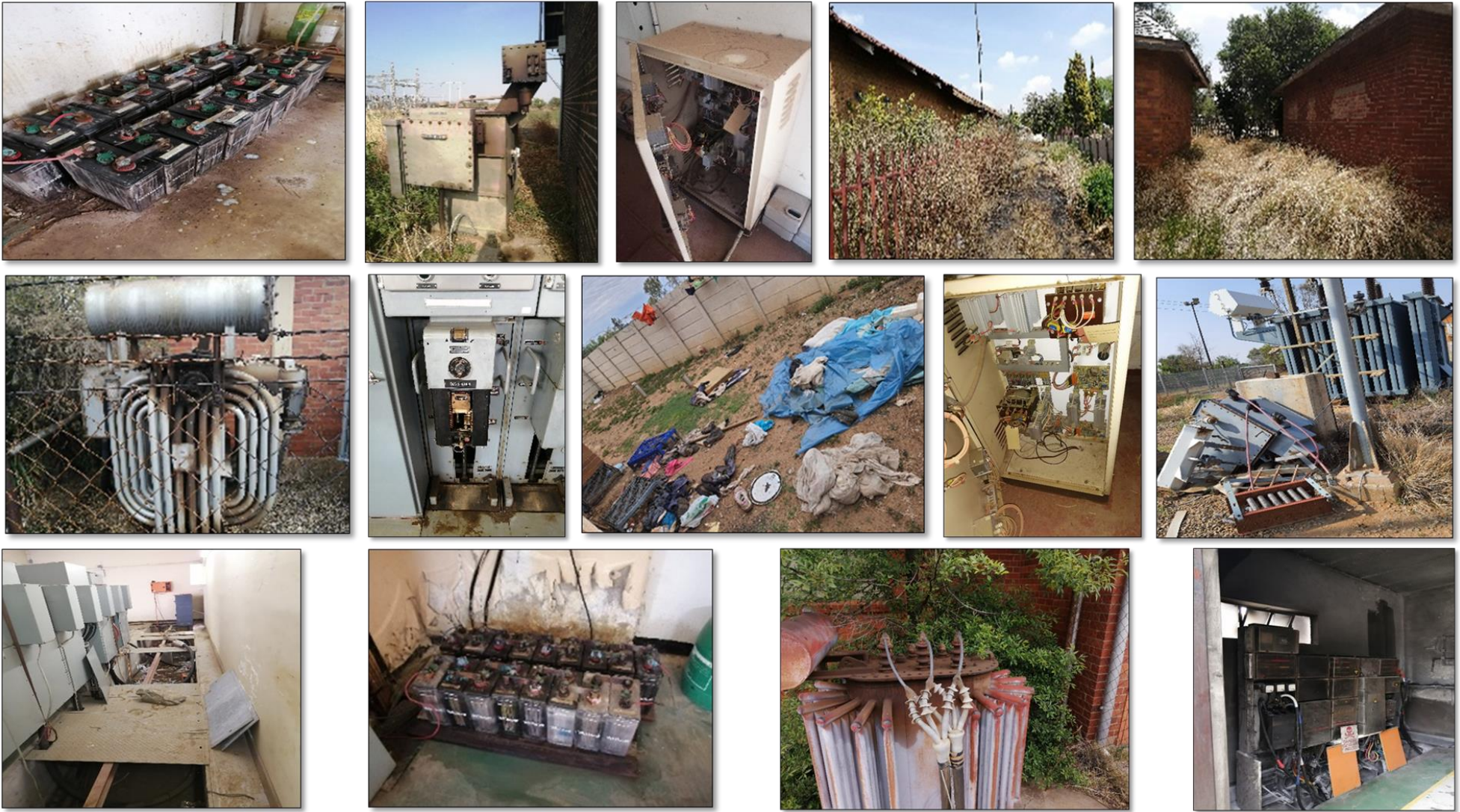
Figure 6-1: Condition Assessment Site Inspection Pictures
